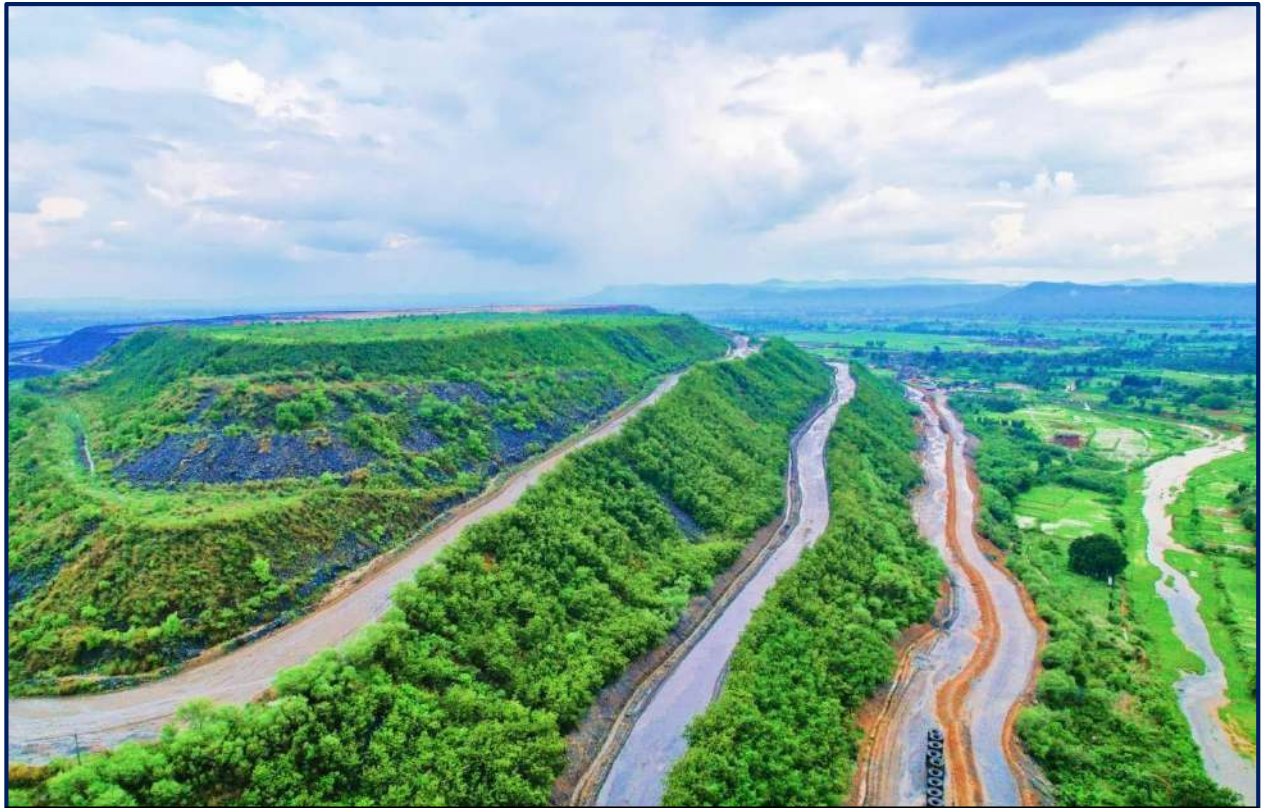
Drone View of Overburden Dumping Plantation Site
