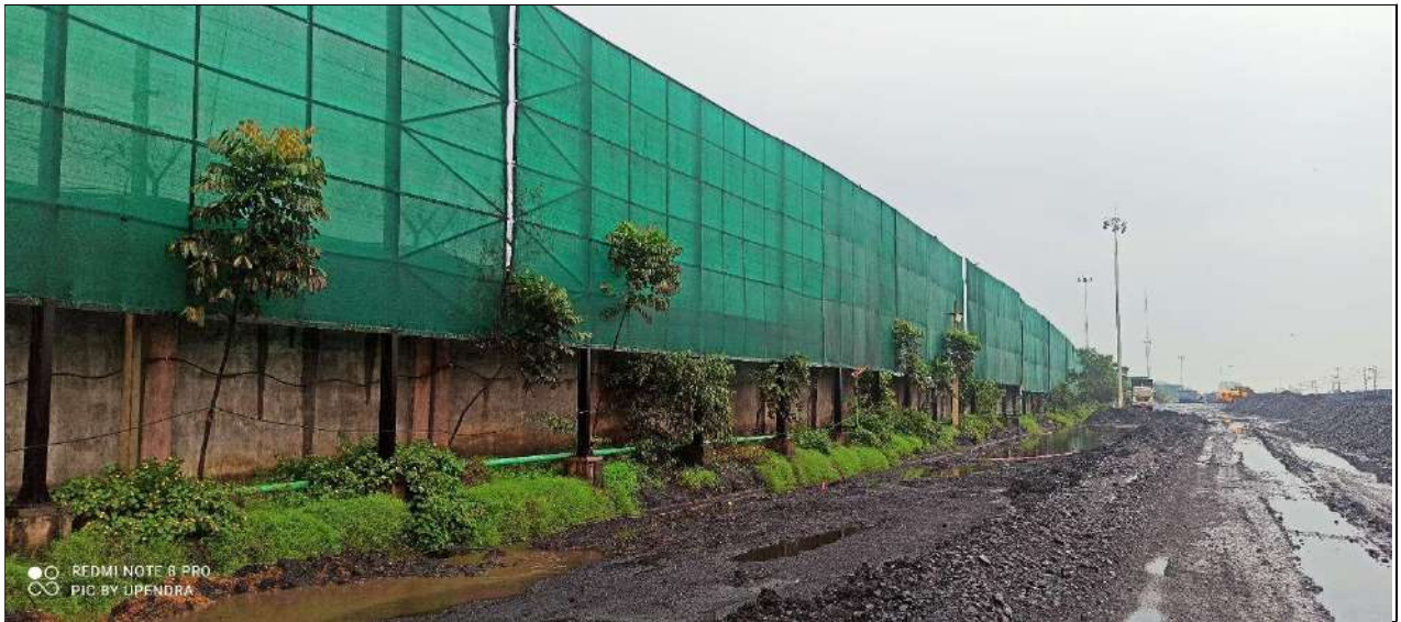
Photographs of Boundary wall with 20 ft. windscreen
