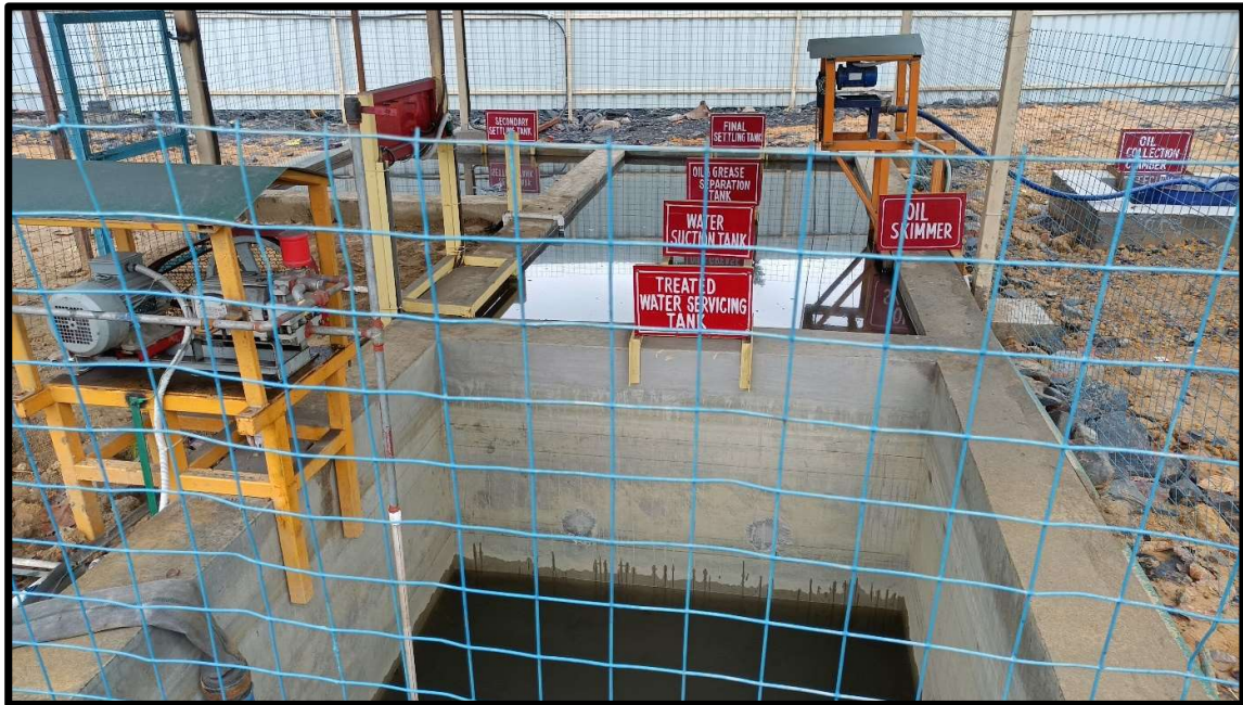
Picture : Oil & Grease Pit at Workshop
