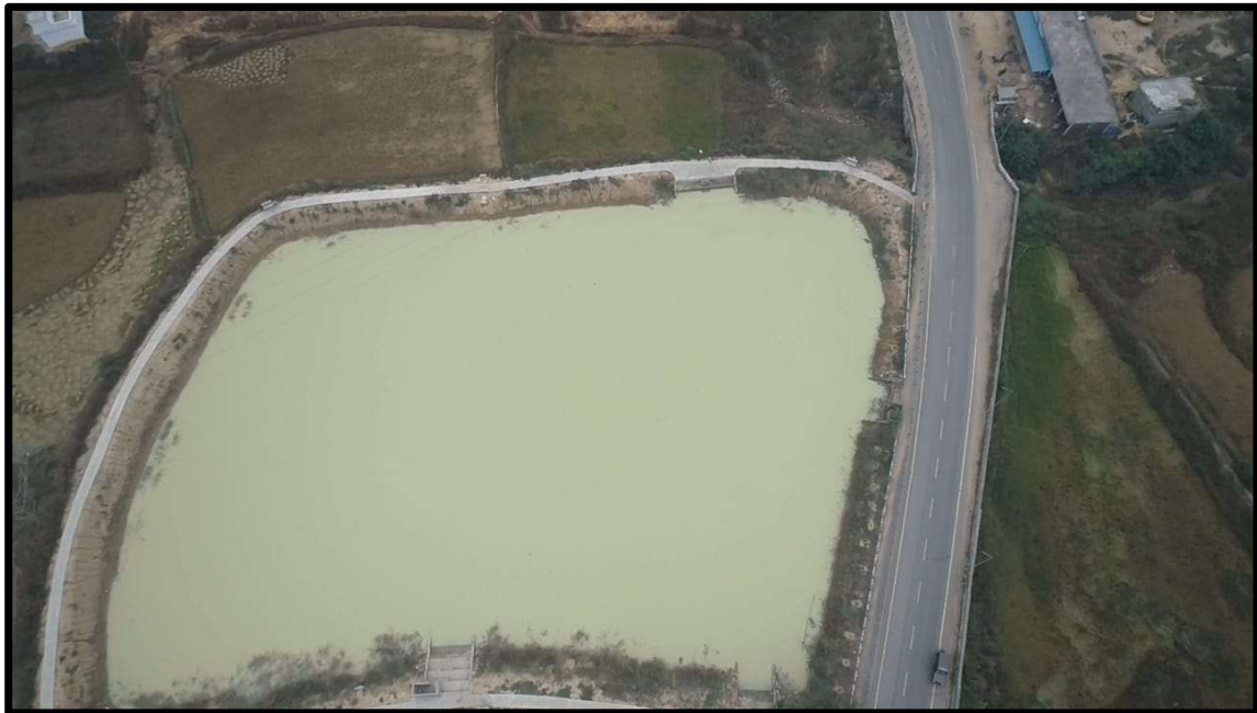
Picture: Pond De-siltation work at Salhepali Village
