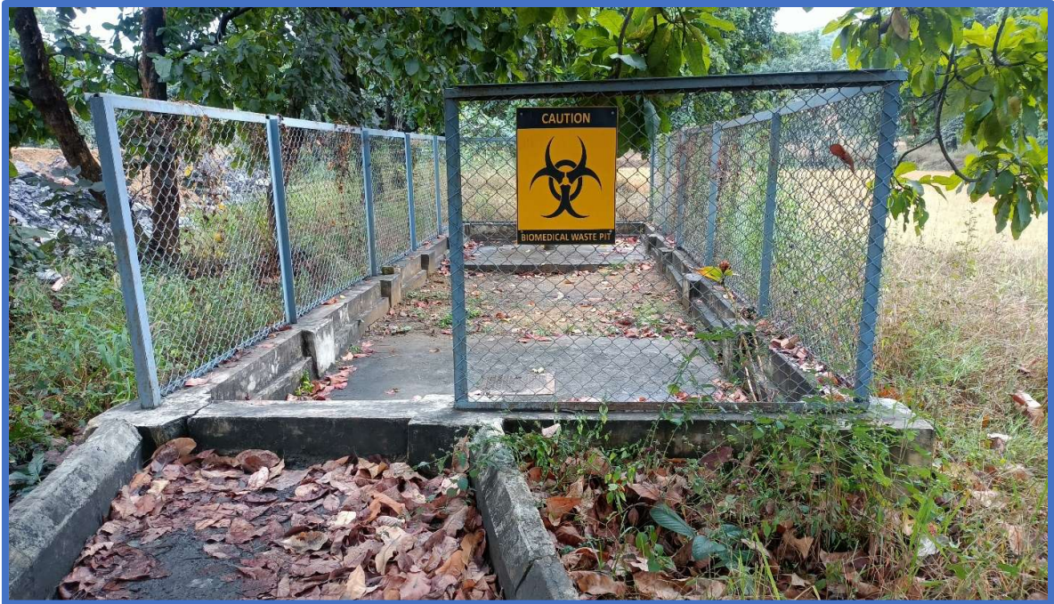
Picture: Underground pit for Medical waste Management
