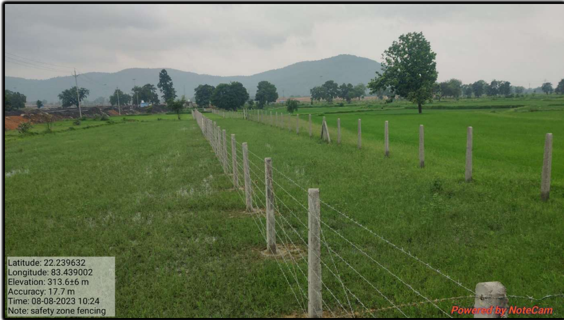
Picture: Safety Zone Fencing work in progress
