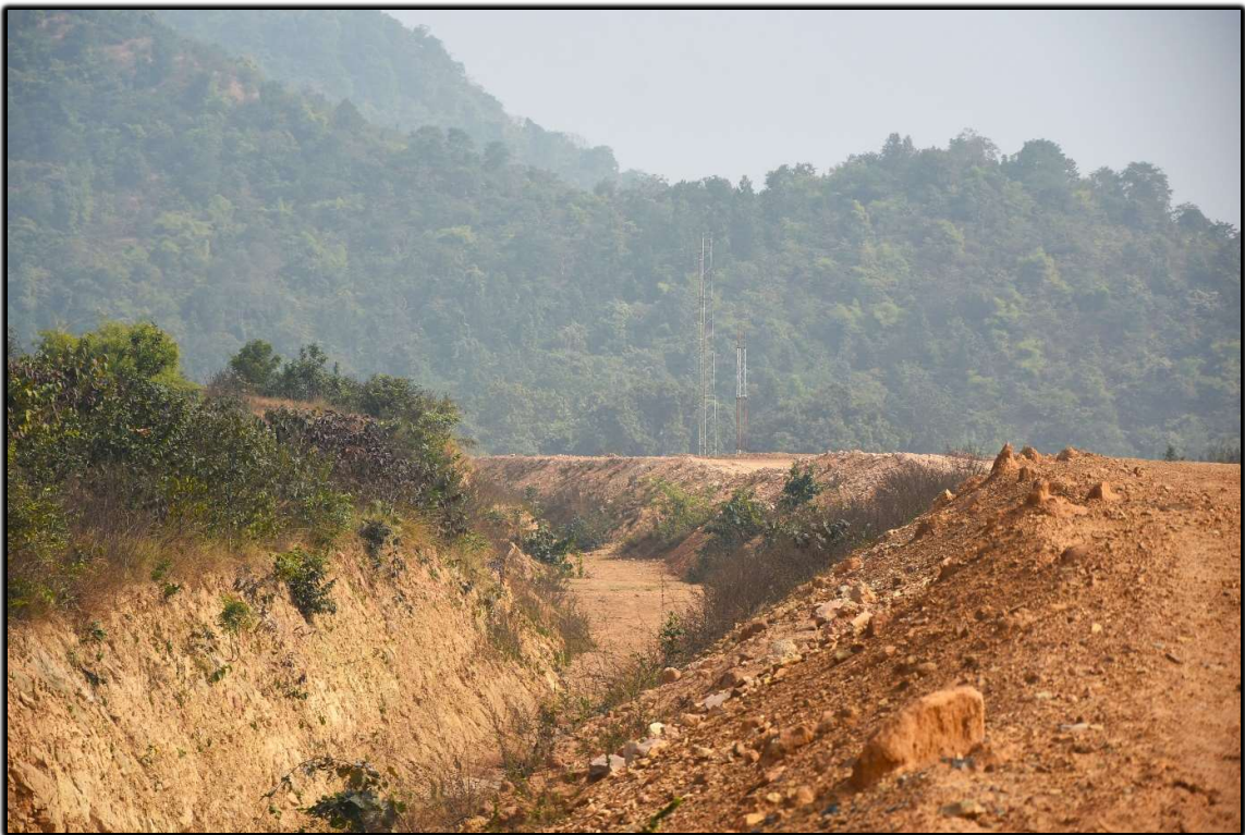
Picture: Construction of Garland Drain along the mine boundary i/p
