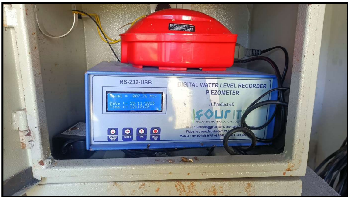
Picture: Piezometer Installed at NTPC TLCMP
