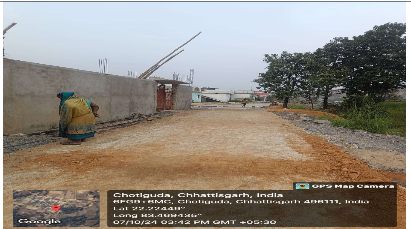
Construction of CC Road at Nayarampur Village.
