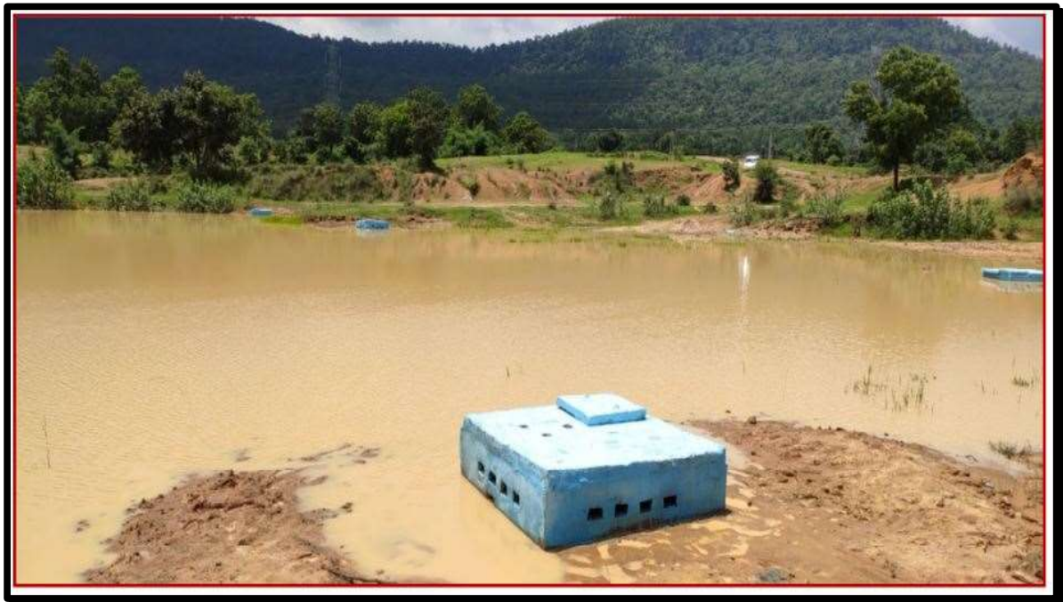
Picture: Ground Water Harvesting Structure
